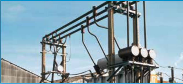
GASLINK® SF 6 insulATED busbar system
