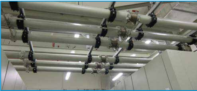
GASLINK® SF 6 insulATED busbar system
